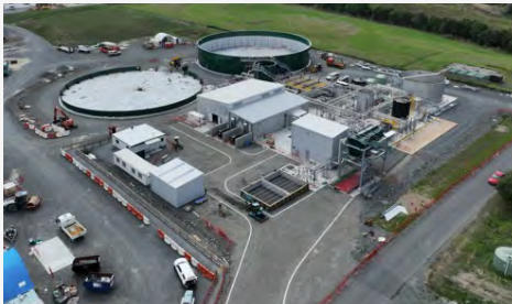
Hautapu site under construction – March 2025
