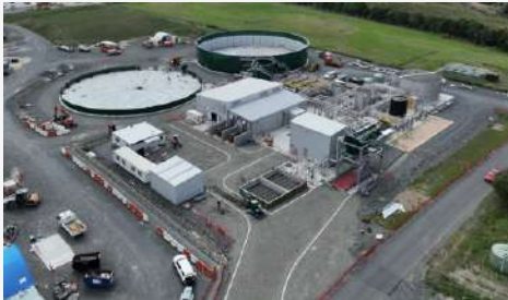
Hautapu site under construction – March 2025
