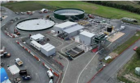
Hautapu site under construction – March 2025
